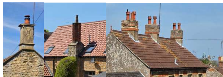
Figure 23: Examples of local chimney types
