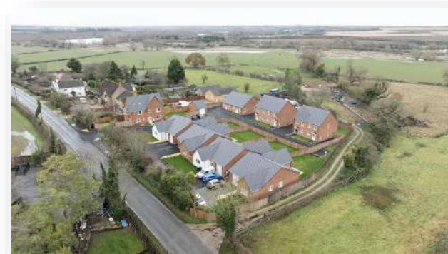
Figure 10: Howards Way rural exception site
